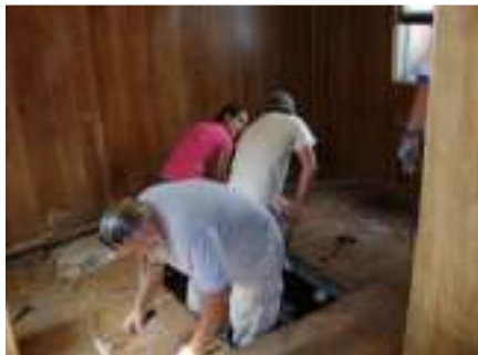
Kingdom Builders installing a new floor for the Arnett Family.
